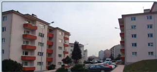
SEEBRIG Accommodation Area
