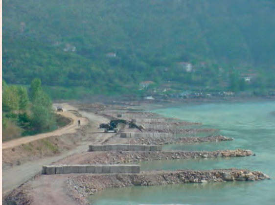
Works to protect the river bank from degradation
