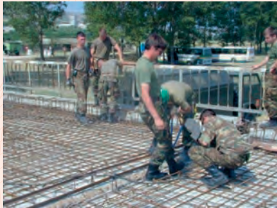
Construction of the bridge deck
