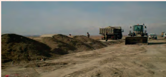
Construction of a protective berm inside “KAIA”
