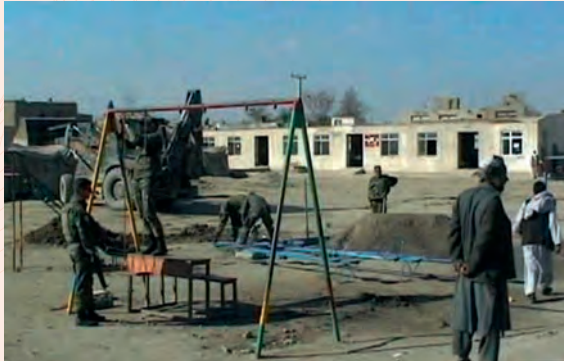
Construction of a playground
