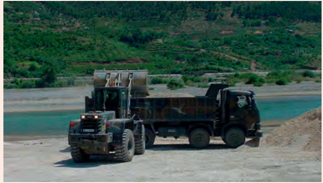
HEPSEC Engineers at work
