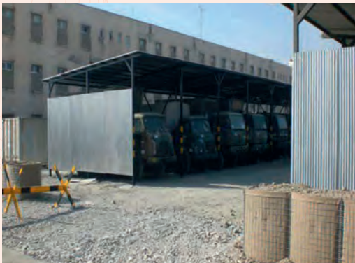
New shed construction at camp "INVICTA"
