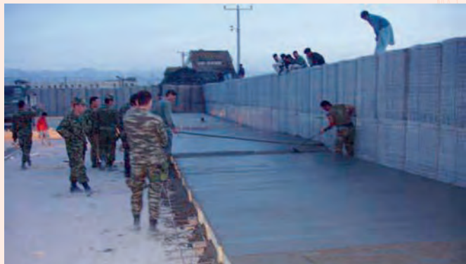
Concrete-pad construction at camp "INVICTA"
